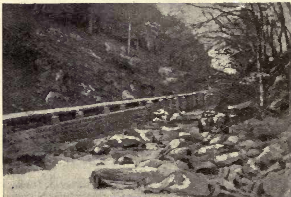
FIG. 4.—PIPE LINE FROM WEIR TO TURBINE HOUSE.
