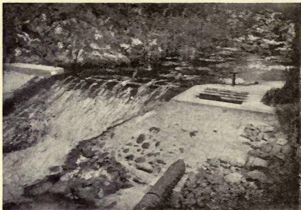
FIG. 3.—WEIR ON SMALL STREAM FOR HYDRO-ELECTRIC PLANT.
