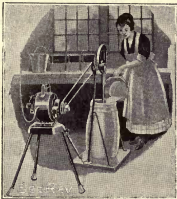
FIG. 32.—ELECTRIC MOTOR DRIVING A CHURN.
